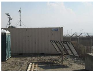
Figure 2 - Solar Stik System powering RFID Interrogator in an Afghani truck yard
