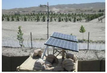
Figure 7 - Solar Stik System powering RFID Interrogator at a convoy rest stop
