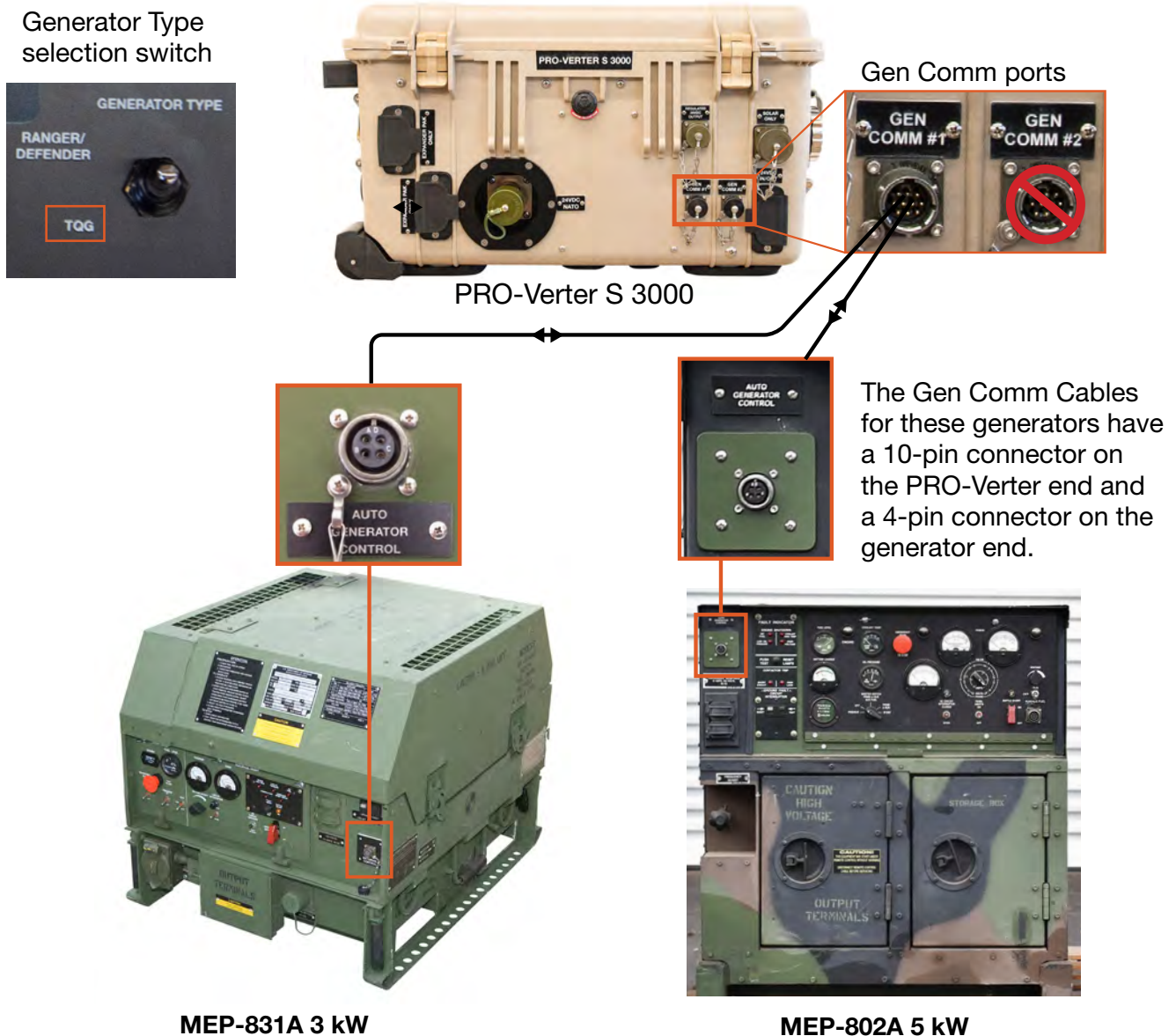
Figure 29. MEP-831A and MEP-802A Gen Comm Cable connections
