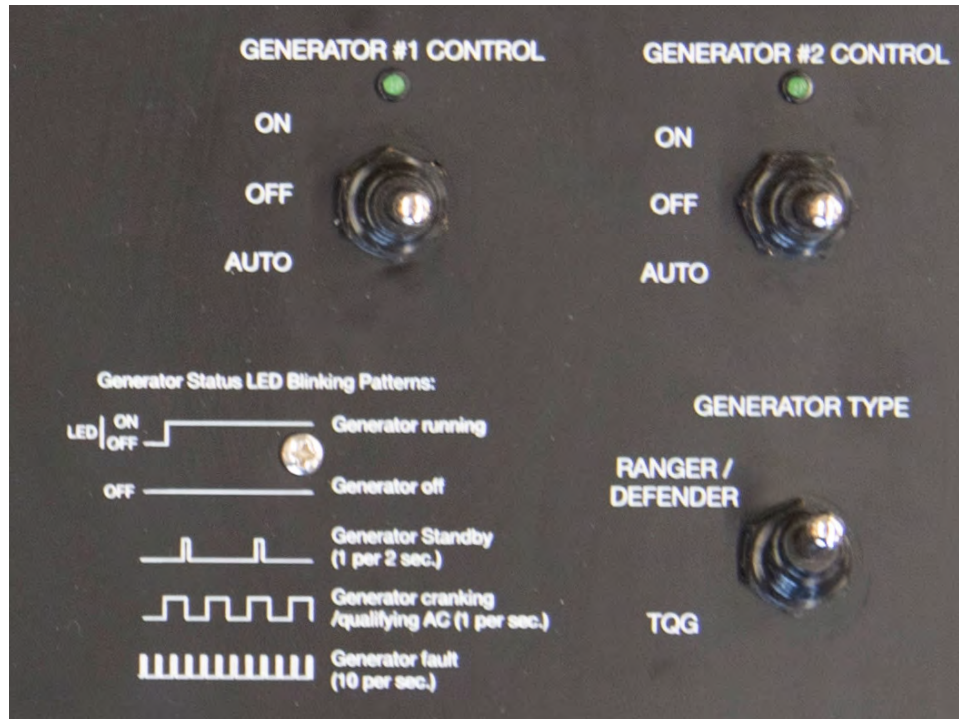
Figure 40. Generator Mode Control Switches and LEDs
