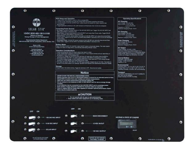
LED associate with breaker/switch will illuminate when switch is toggled ON and circuit is active.
