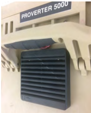
Figure 19. Louvered vent cover
