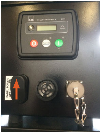
Figure 15. Generator control panel
