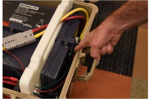
Figure 16. BMS LED indicator light
