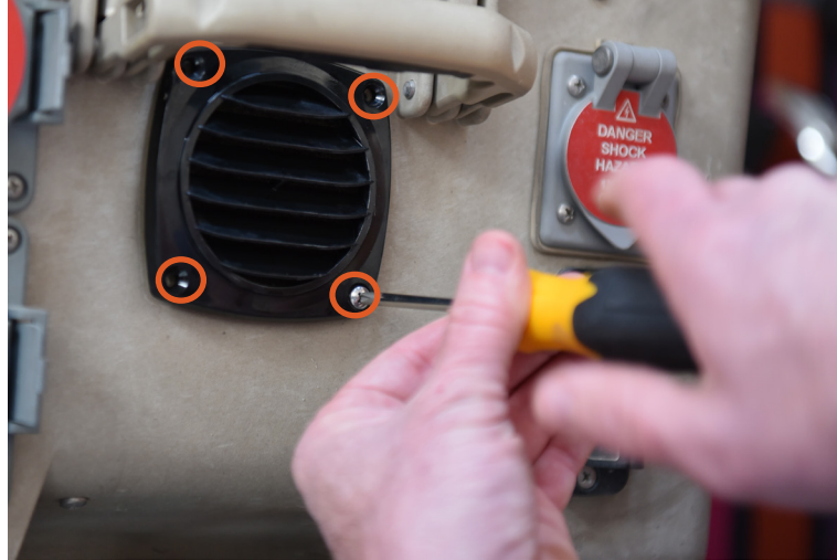
Figure 9. Removing fasteners from louvered vent cover (original version)
