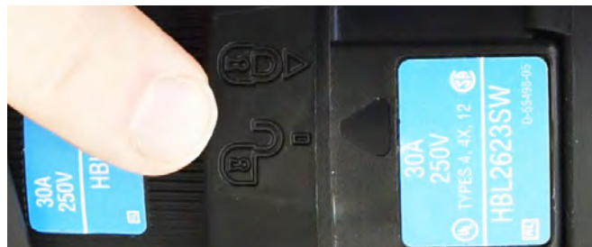
Figure 29. Hybrid Power System bypass twist-lock connection
