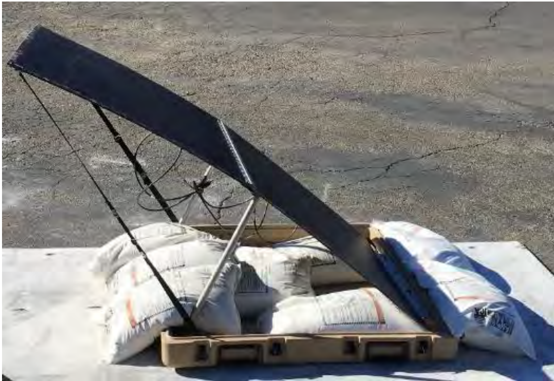
Figure 23. Securing arrays to ground with sandbags
