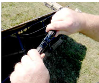
Figure 21. Disconnecting cables and unlocking panels from rack
