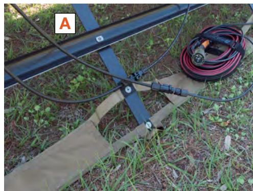
Figure 11. Loose solar panel lead wires (A) versus tucked away, protected wires and H4 PV connectors (B)
