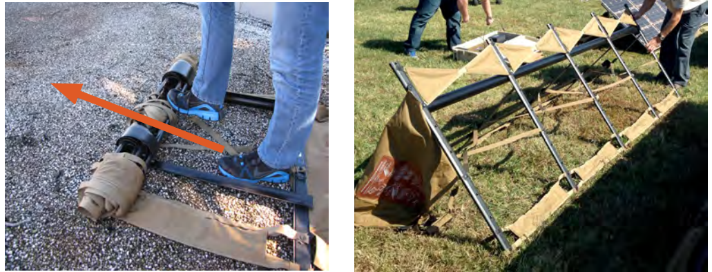
Figure 6. Unrolling and standing up panel support rack
