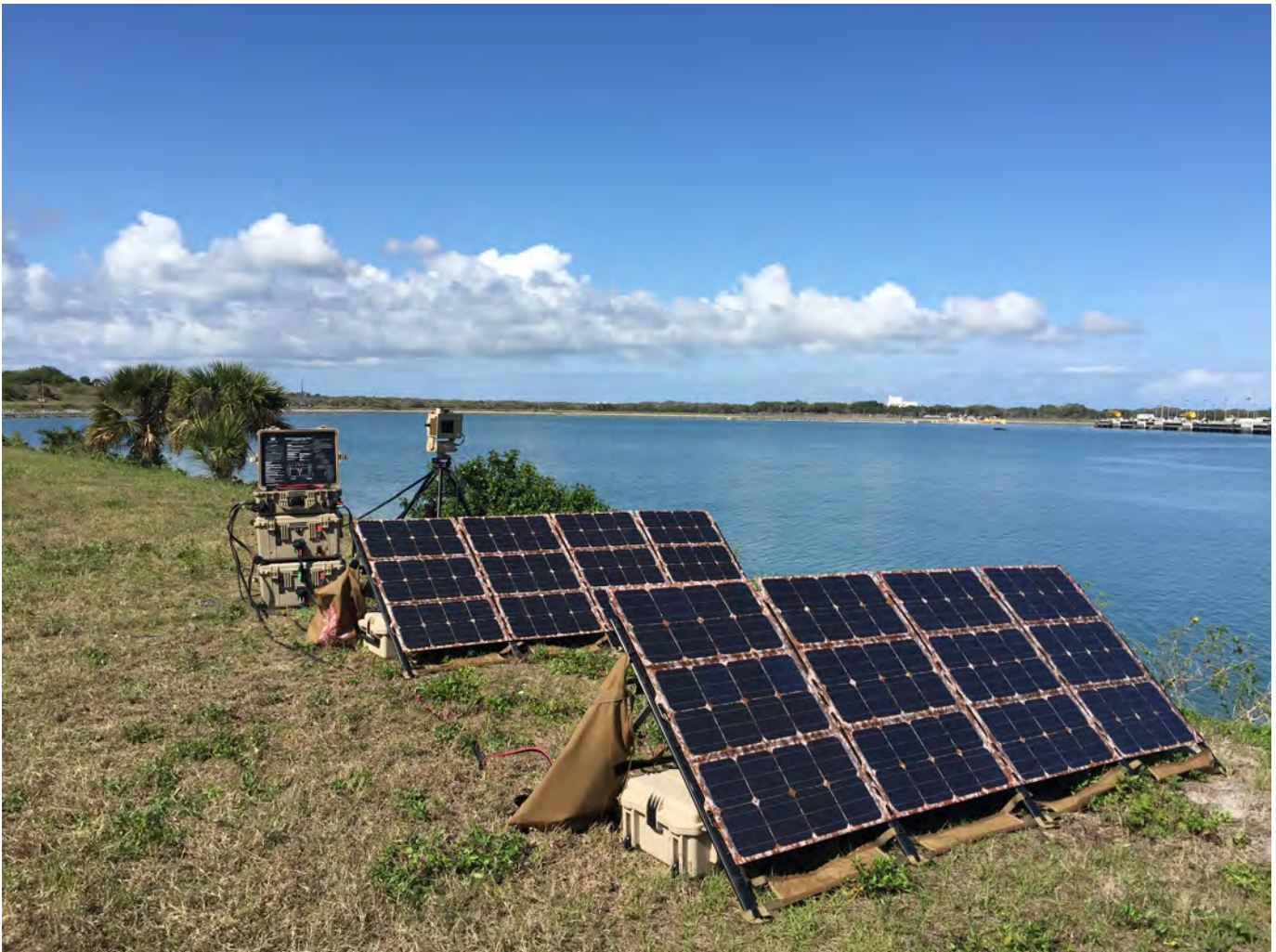
Figure 1. Solar Arrays, Power Hub, and Expander Paks supporting a sensor
