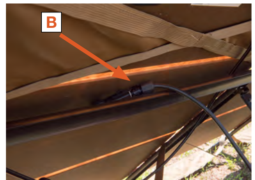
Figure 11. Loose solar panel lead wires (A) versus tucked away, protected wires and H4 PV connectors (B)
