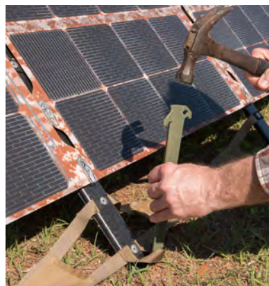
Figure 16. Securing PV arrays with stakes
