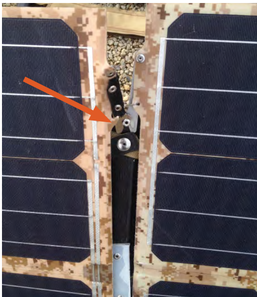
Figure 18. Bent or broken catches and latches along side of the PV panel
